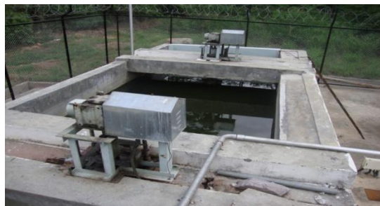
Figure.11 Surface Aerators In The Aeration Tank At CFTRI
