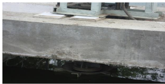
Figure. 9 Immersible Depth Of Impeller Into The Effluent (Stage-Ii)
