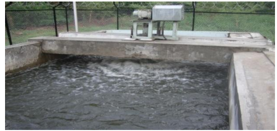
Figure.8 Immersible Depth Of Impeller Into The Effluent (Stage-II)
