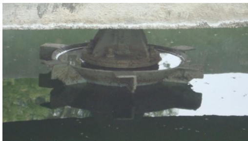
Figure. 10 Immersible Depth Of Impeller Into The Effluent (Stage-Ii)
