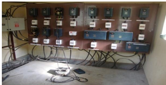
Figure. 3 Connection Of Motor Frequency Converter In The Motor Control Room
