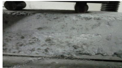
Fig. 1: Typical Beam Specimen Showing First Crack During Loading
