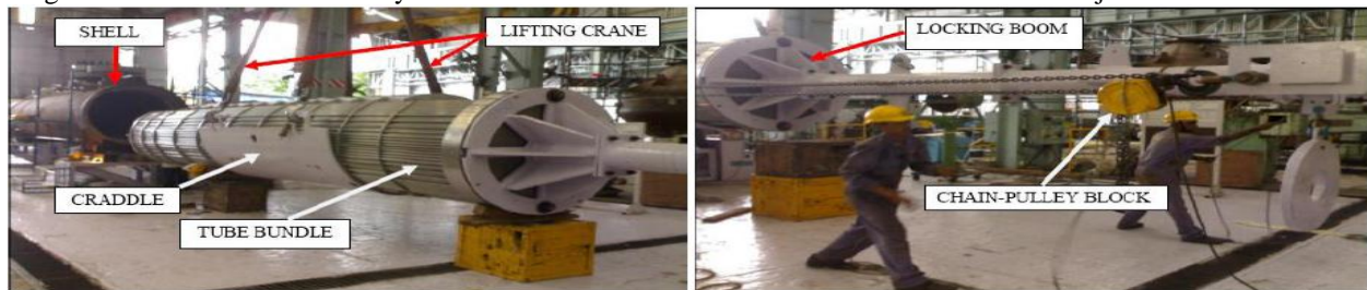
Fig.1-Pictures showing manual tube bundle insertion activity
