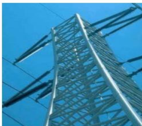
(a) Composite Transmission Tower
