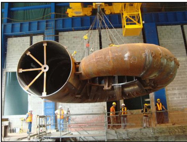
Figure 19. Process of assemblage of the spiral chamber
