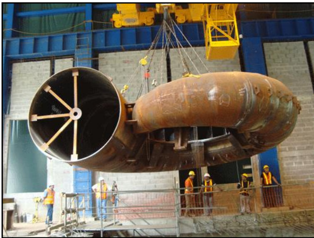
Figure 19. Process of assemblage of the spiral chamber
