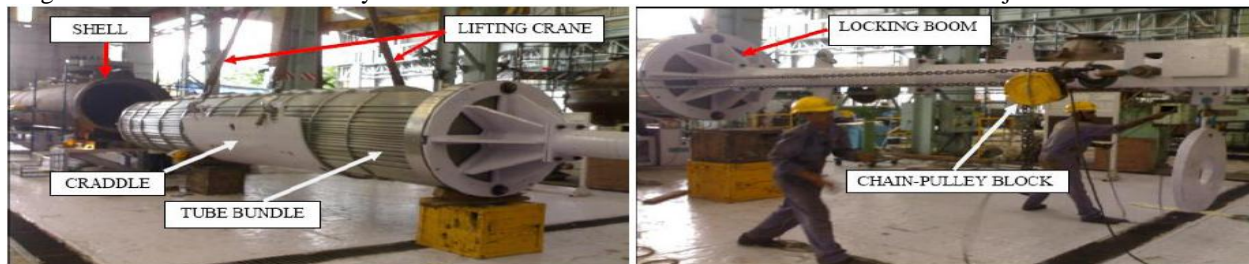
Fig.1-Pictures showing manual tube bundle insertion activity
