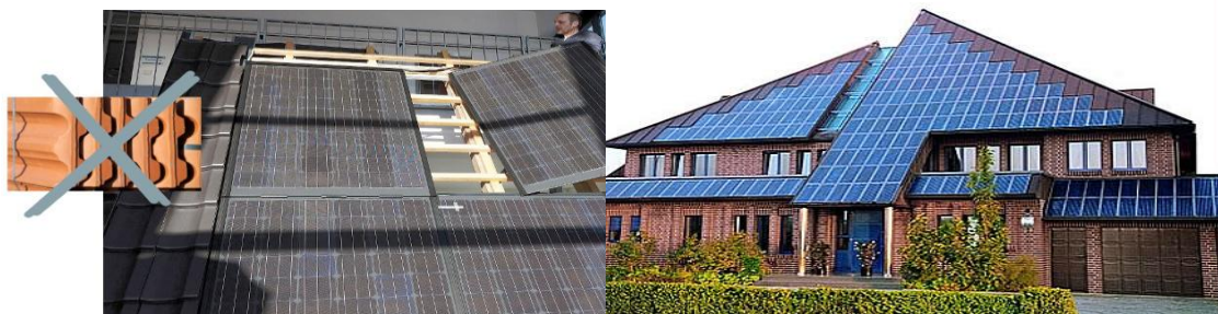
Figure 4: Replacing tiled roofs with solar panels.
