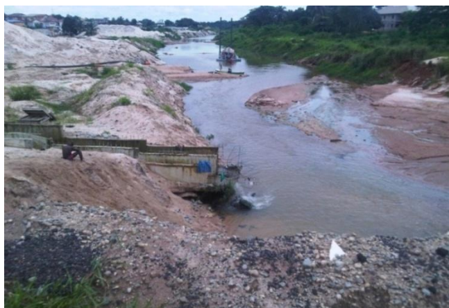
Plate 1: Erosion at Discharge Point
