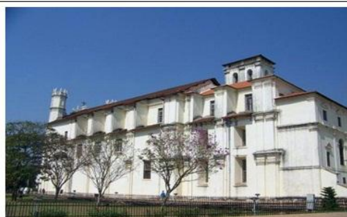
Fig. 2. Convent and Church of St. Francis Assisi
