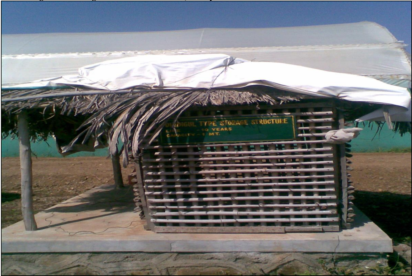
Figure 2: Dindigul onion storage structure
