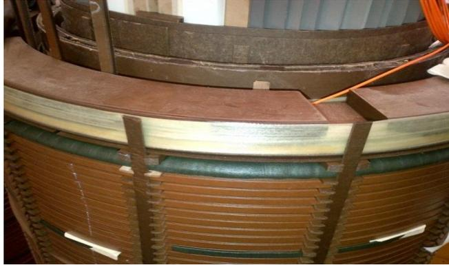
Figure 4a Location of probes in the power transformer
