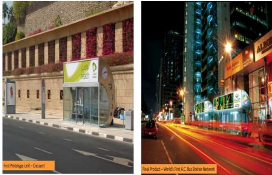
Figure 41: night view of the Air-Conditioned Bus Shelter
