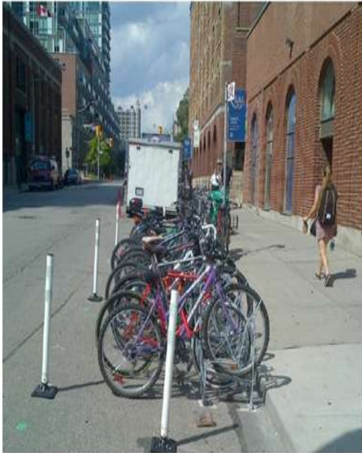
Figure 37: Bolting racks corral
