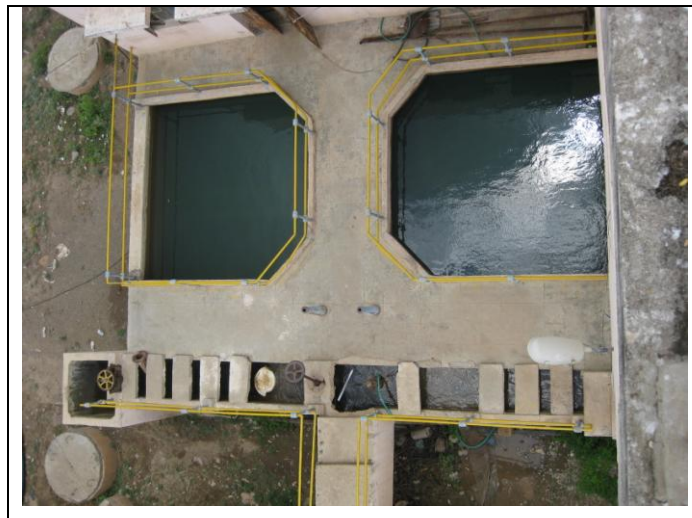
Fig No.2 sand Filtration
